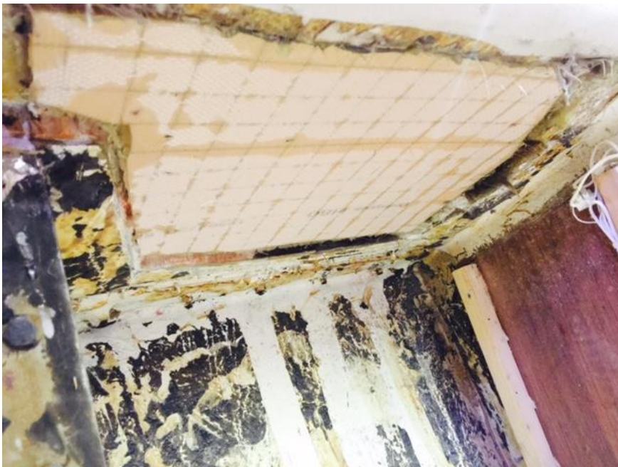
Figur 9 Distansmaterialet fast i taket
